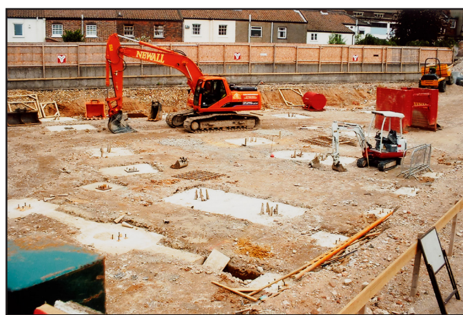
Digging the foundations for SSG in 2006
